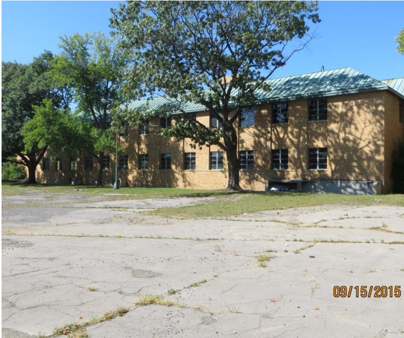
Partial view of building's east side
