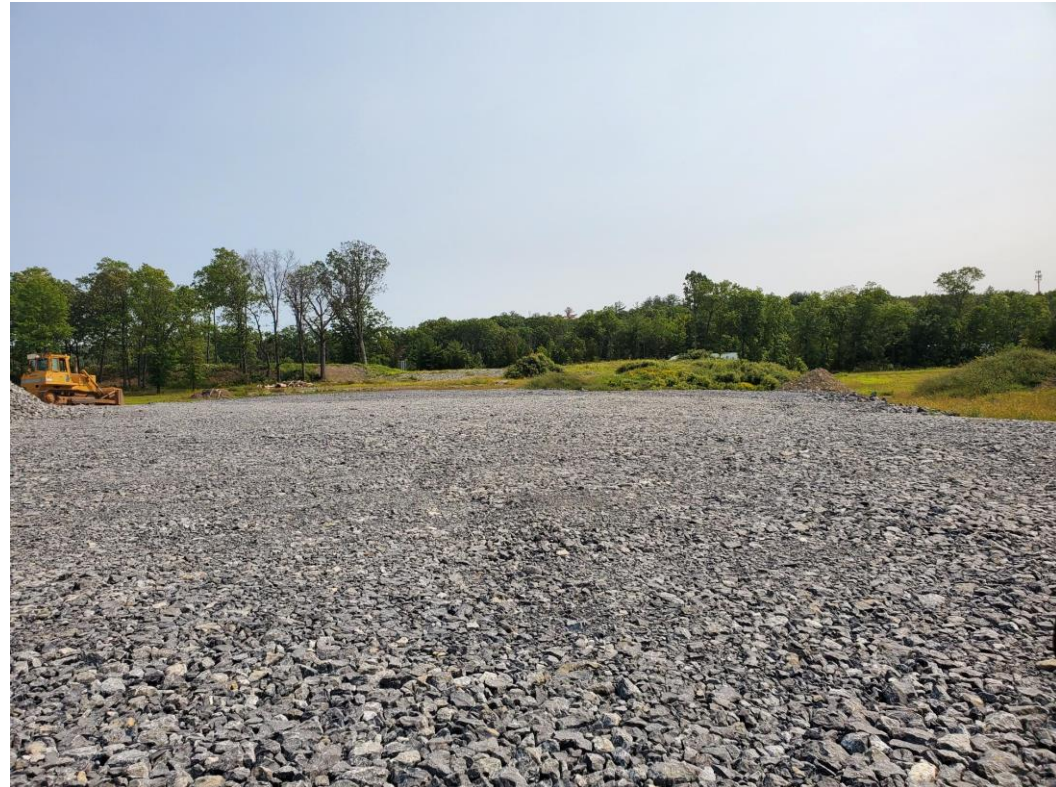
Site at rear
