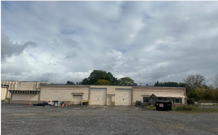
Multiple Overhead Doors
