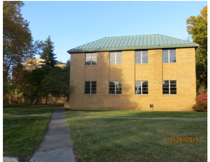
View of south side
