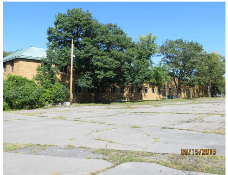
View from east lot
