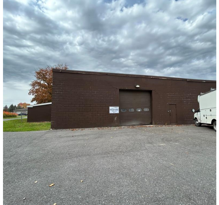
Drive-in Door / Rear Entrance to Warehouse – Tenant 2
