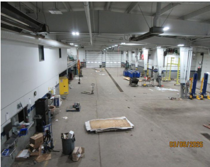
Interior – shop area
