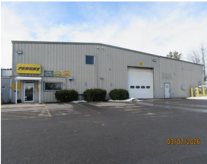
Customer entry – east side
