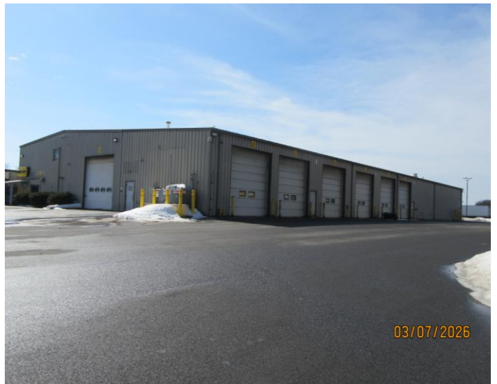
Nine total OH drive-in doors
