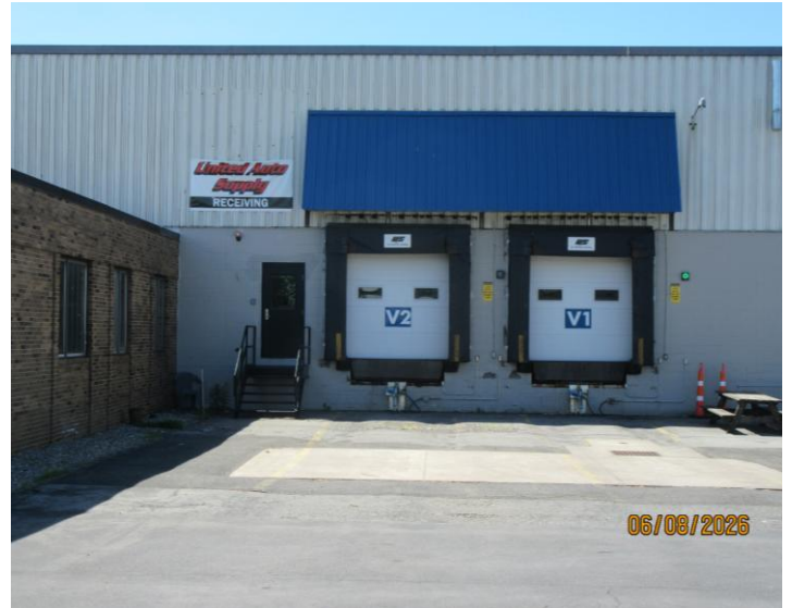
Loading docks with levelers
