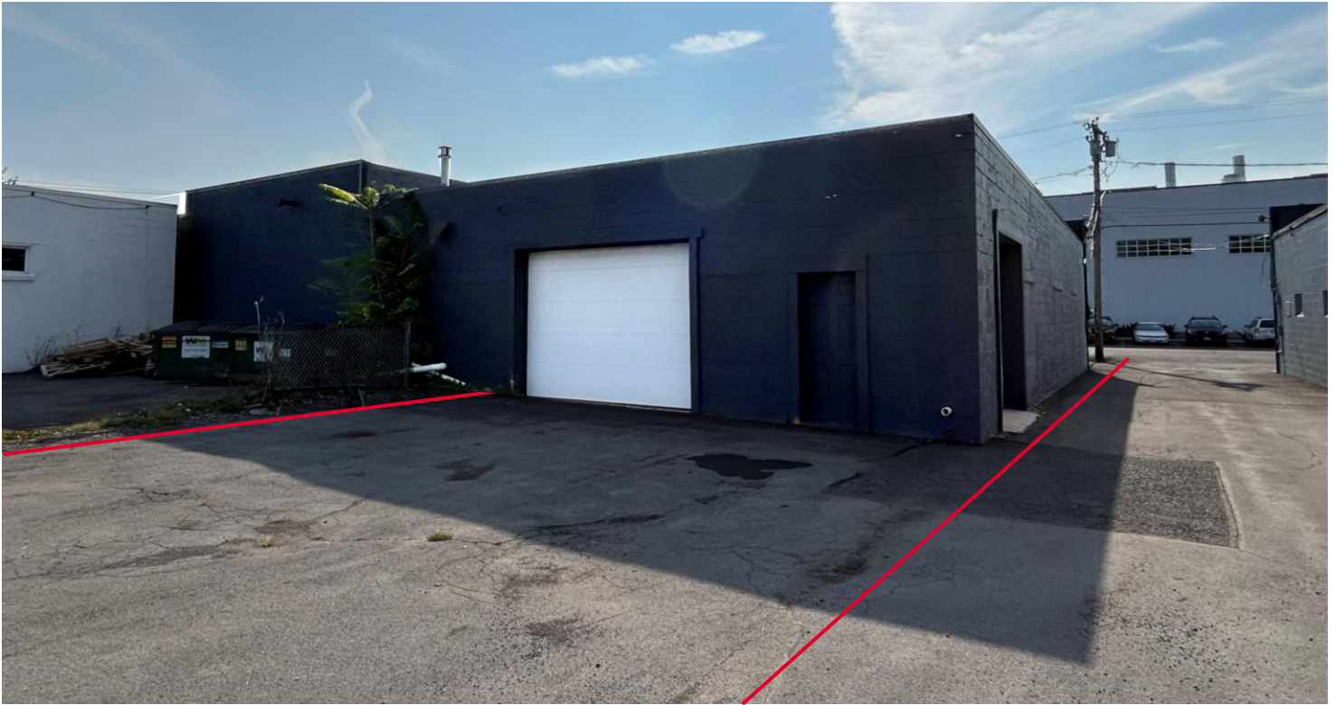
Property line is tight to the building, dumpsters belong to neighboring building
