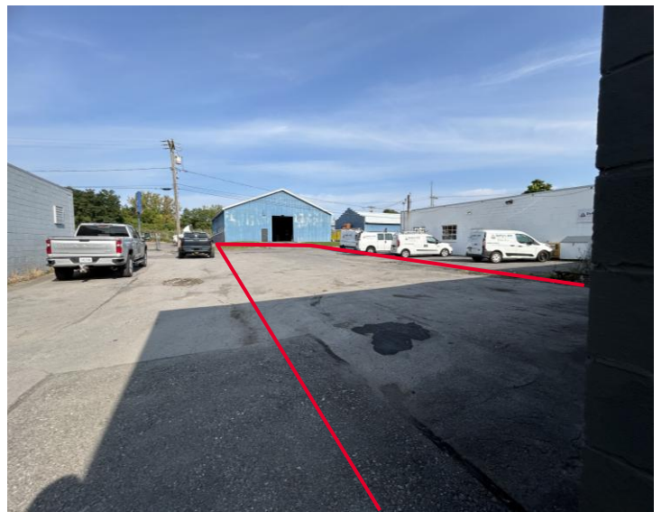
Parking area in rear of building
