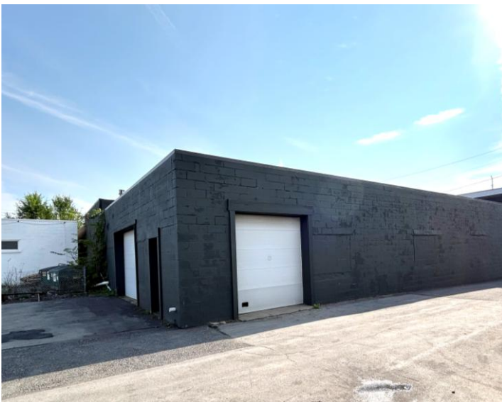
Two drive-in overhead doors at rear
