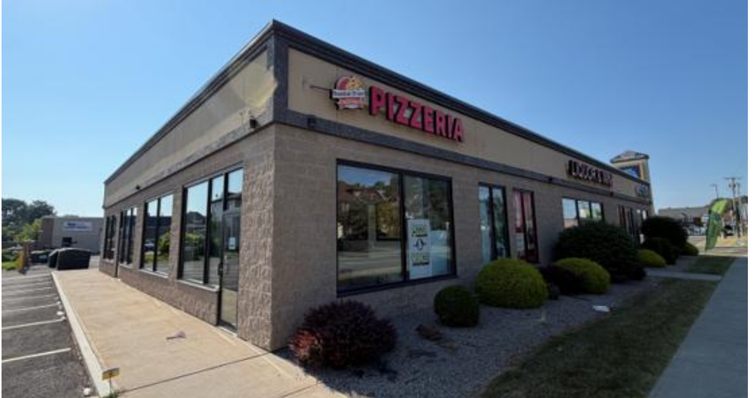
Geddes Street frontage
