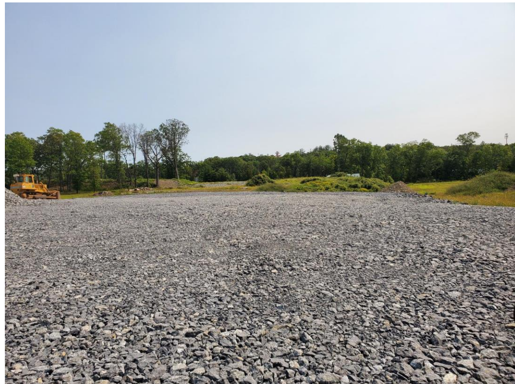
Site at rear
