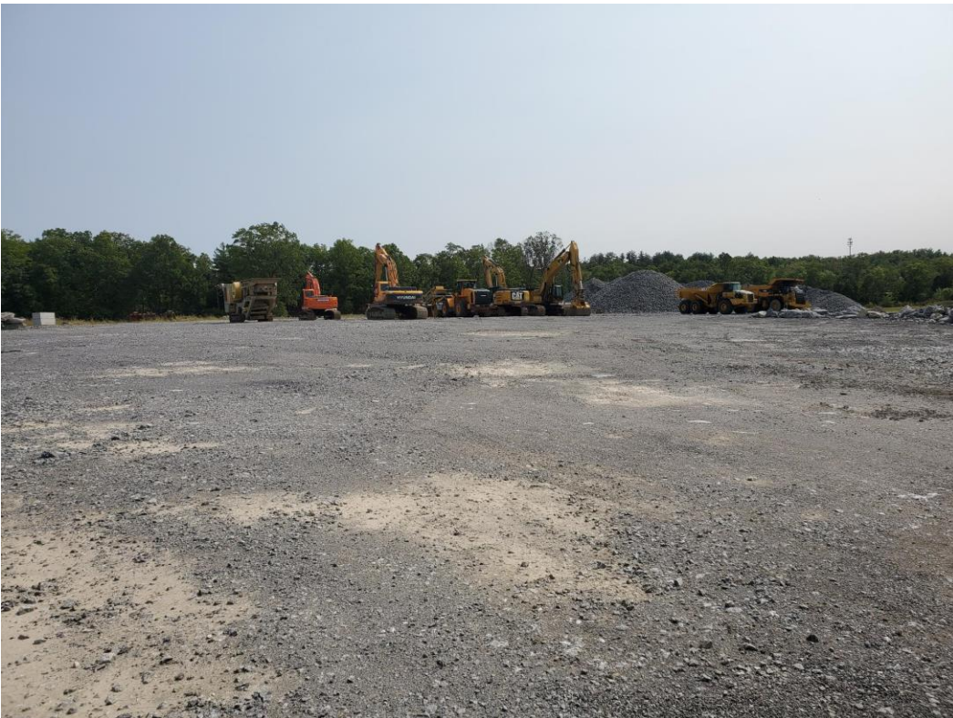
Site with equipment
