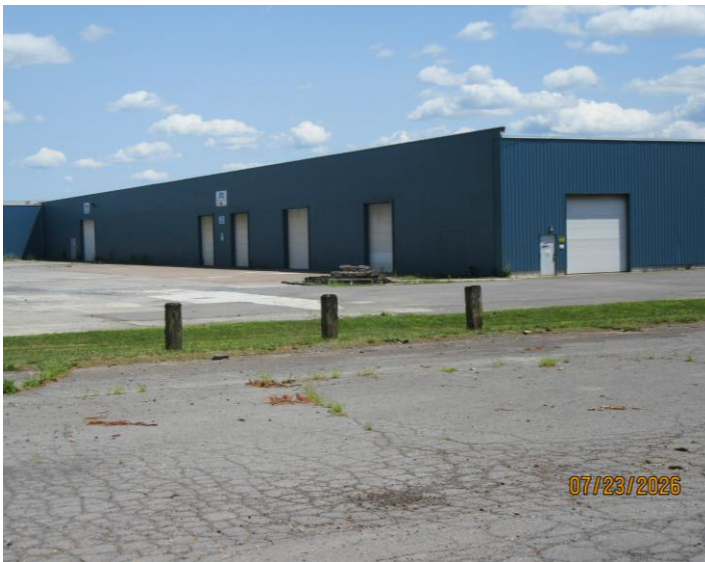
Six (6) drive-in doors (14' high)
