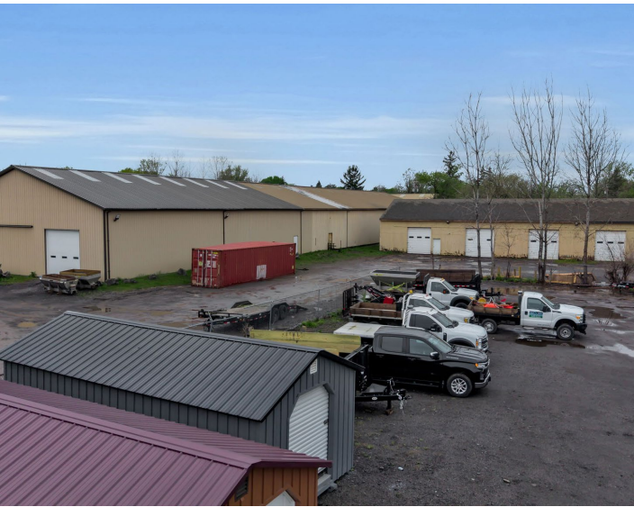
Rear Warehouse Building
